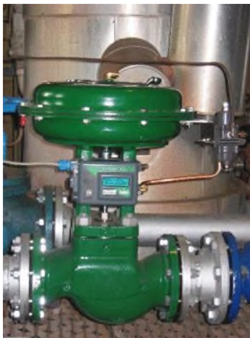
8.29-rasm. Rostlanadigan klapandagi membranali pnevmatik yuritma
