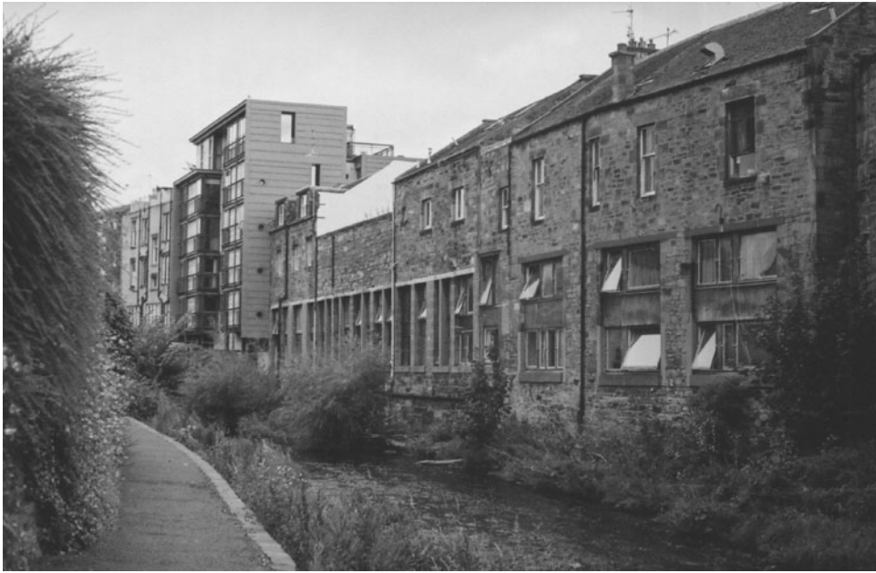
Figure 13.5 Water of Leith Walkway, Edinburgh, Scotland (Photograph by author, 2007)
