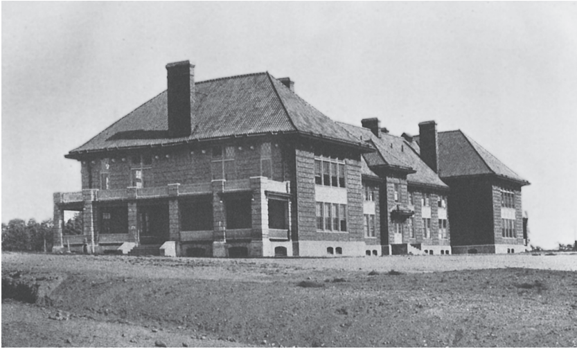
FIGURE 11.1. Cottage No 4—Group III, one of the not-yet-massive residences that housed, in total, a population of patients approaching 4,000. From Seventeenth Annual Report of the State Hospital at Kings Park to the State Hospital Commission for the Year Ending September 30, 1912 , plate between pp. 22 and 23.
