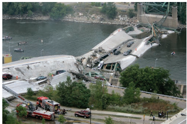
The collapsed freeway bridge over the Mississippi in Minneapolis in August 2007.
