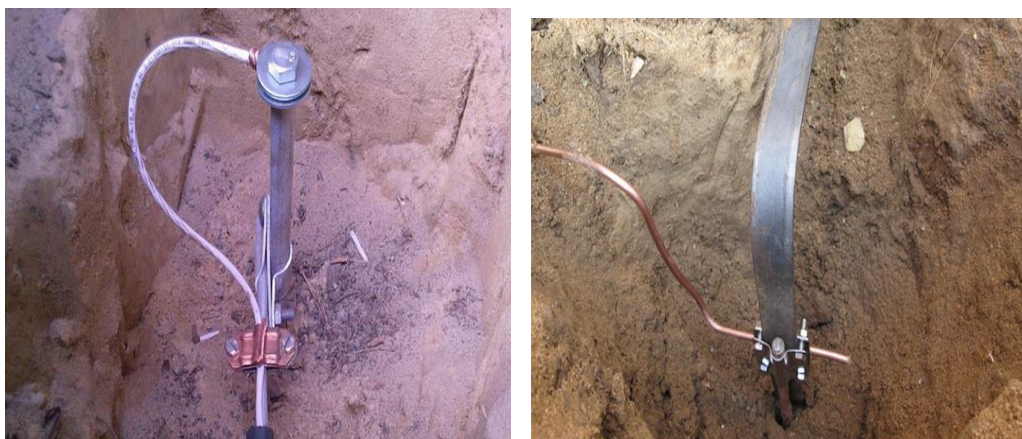
3.16 – rasm. Vertikal elektrodni transheyaga o‘rnatish qurilmasi
