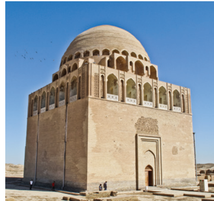
Plate 20. Sanjar's vast mausoleum at Merv. Its ingeniously engineered double dome, visible at a full day's journey from the capital, launched a movement that created prototypes for such domes in the West. ■ Peretz Partensky/Langton Labs.
