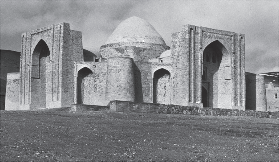
Figure 14.6. Tomb of Ulughbeg at Ghazni in Afghanistan. This and other Timurid structures deeply influenced architects in Mughal India and Saffavid Iran, even serving as models for the Taj Mahal. ■ Josephine Powell Photograph, courtesy of Special Collections, Fine Arts Library, Harvard University.
