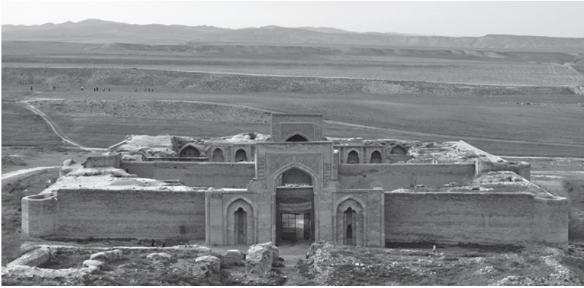
Figure 12.1. In spite of their nomadic background, Seljuk rulers eagerly embraced commerce, as is reflected in this enormous caravanserai they erected on the Nishapur–Merv road. ■ Photo by Harry Reid, London.
