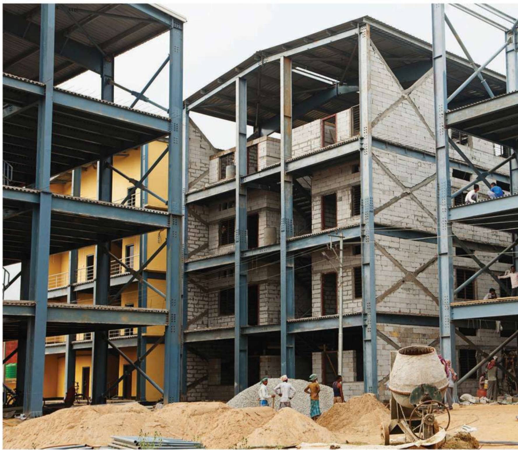
▲ ONCE COMPLETED, INDIA'S LARGEST IMMIGRATION DETENTION CENTER WILL HAVE A CAPACITY OF 3,000
