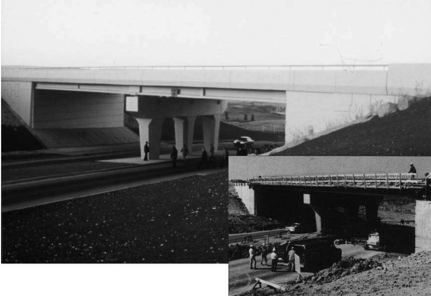
FIGURE 9.34. Beddington Trail Bridge in Calgary during construction and when open to the public in 1993.
