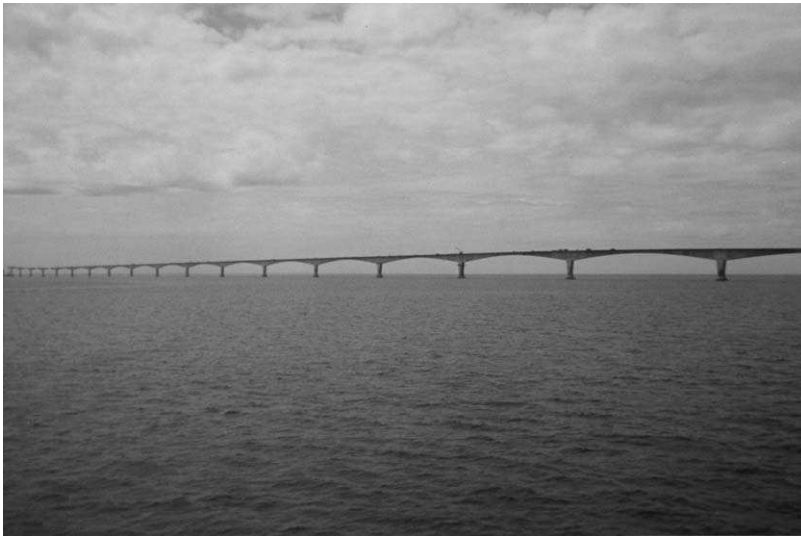
FIGURE 9.54. A view of the 12.9-km ocean-crossing Confederation Bridge, linking Prince Edward Island to New Brunswick in Canada.
