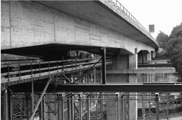
FIGURE 10.26. Versoix Bridge near Geneva, Switzerland. Courtesy D. Inaudi, Smartec.
