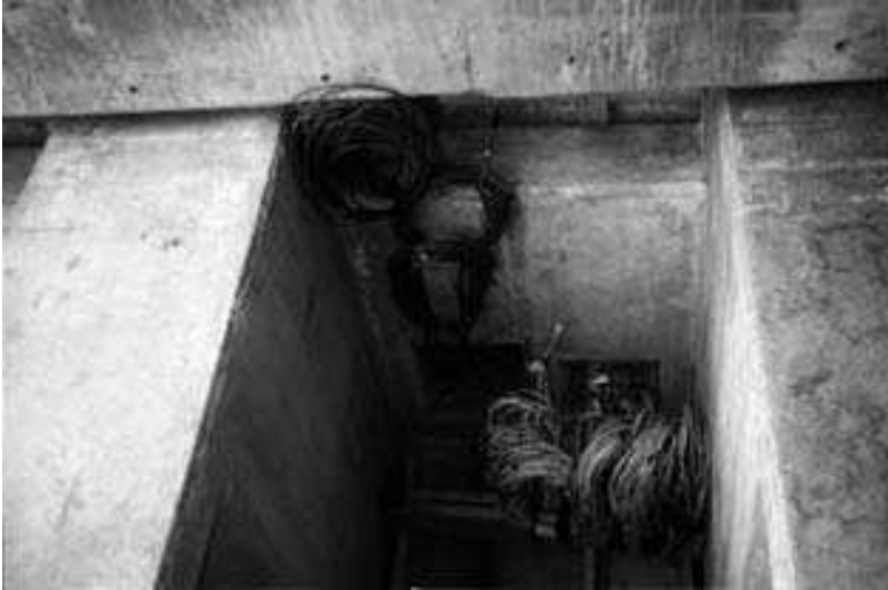
FIGURE 8.9. Example of the special metal housings provided at the egress point for the fiber optic sensor cables used on the Confederation Bridge. These housing protect the optical fiber cables during construction (and if necessary, transportation) of the concrete structure. Used with permission, ISIS Canada.
