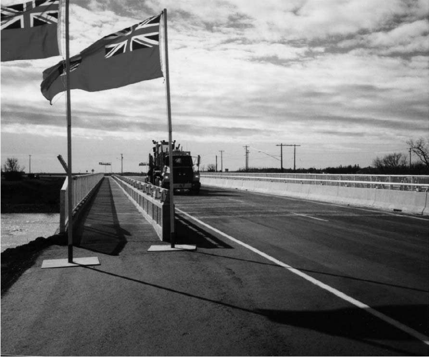
FIGURE 2.5. Taylor Bridge in Winnipeg. Used with permission, ISIS Canada.
