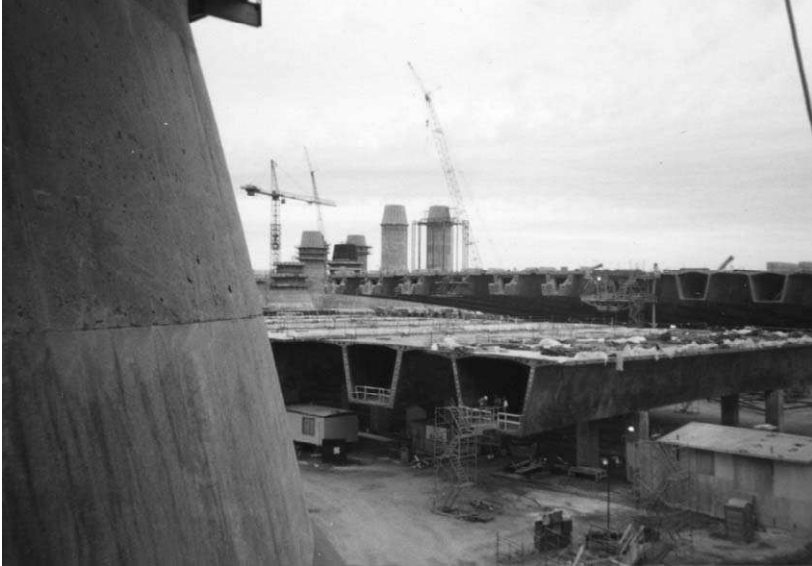
FIGURE 9.55. An overview of the Confederation Bridge component construction and assembly yard.
