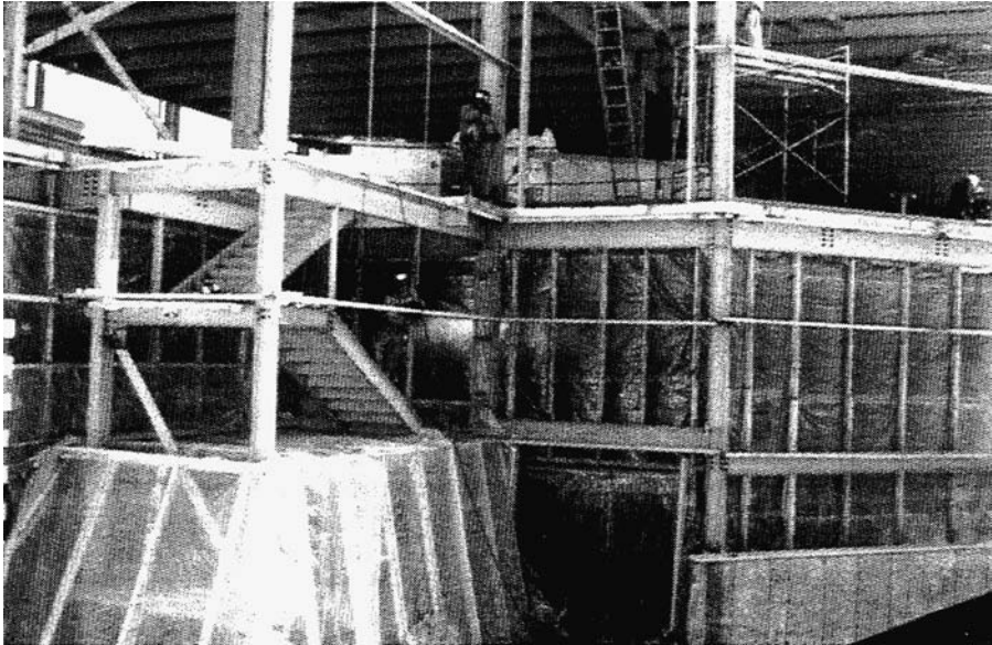
Figure 8.9 Structural steel erection for equipment mezzanine. (Photo courtesy of Gilbane Building Co.)
