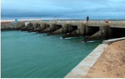
Dam with a flood gate
